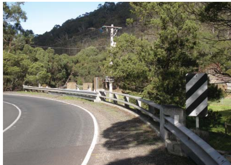
Bridge rail at Grassy Creek on Great Ocean Road (24 years old)
