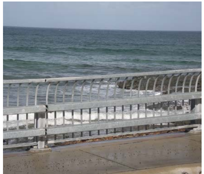
Bridge rail at Smythes Creek on Great Ocean Road (10 years old)
