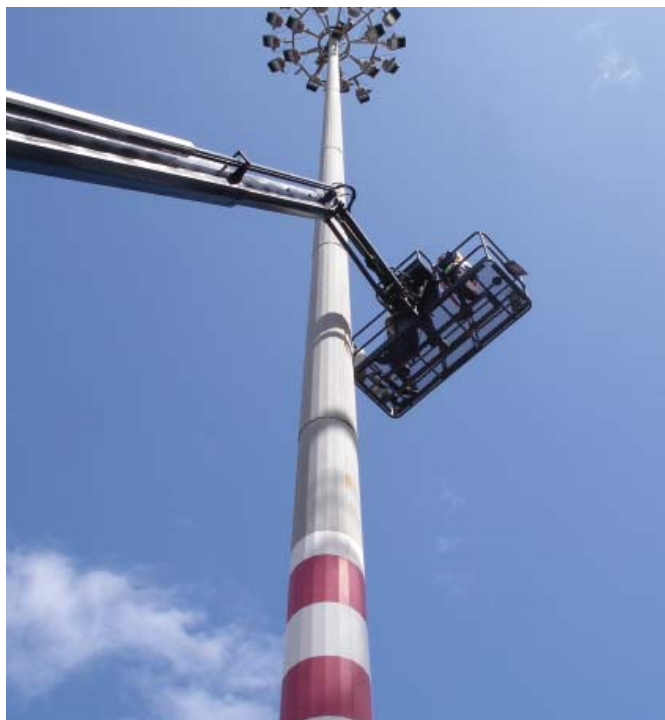
Port of Botany light tower being examined (27 years old)
