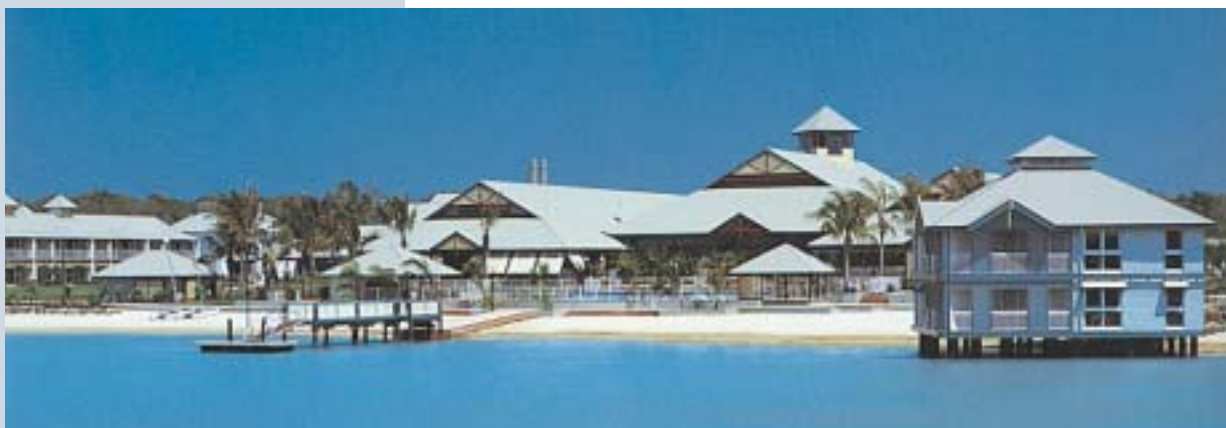
Photo: BHP Steel
