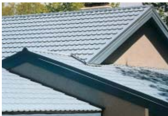
Photo: BHP Steel
