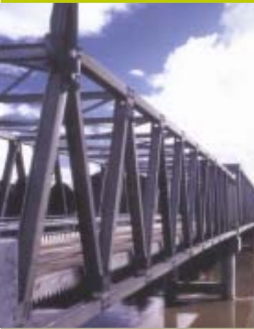
The Ngon Bridge – Laos
