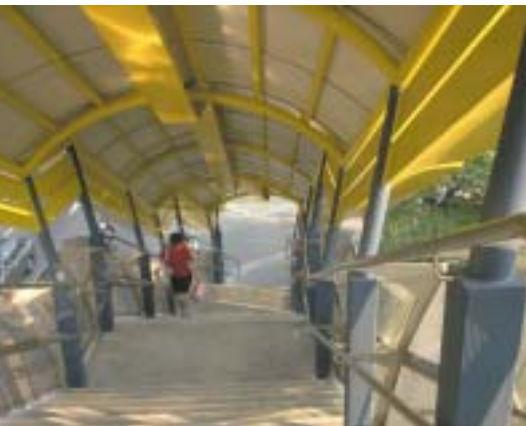
JLN Bukit Timah Pedestrian Bridge
