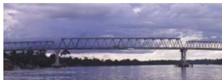
Long Span Truss Bridging
