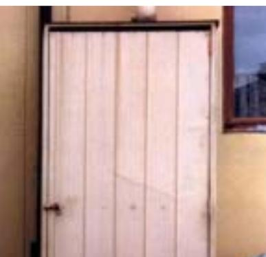
FIGURE 2: Painted galvanized shed and concrete wall showing marked colour differences using the same paint, due to more rapid chalking because of the higher ambient temperature reached on metal.
