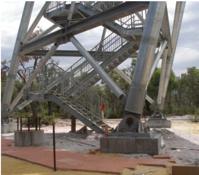
The hinged base of the Leaning Tower
