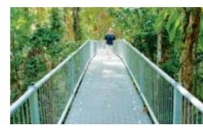
In this context severe steel corrosion is often illustrated as being only at the ocean's edge, in surf or high seas; however the complex environment of this tropical forest includes high salinity, long surface wet time, mould growth, elevated temperatures, and intense UV exposure, all conditions which can contribute to high rates of corrosion within the constant erosion and attack of an undisturbed cycle of life, decay and regeneration.
