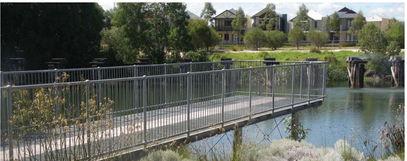
Top: Railway tracks in the Coal Dam Above: Galvanized steel viewing platform
