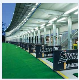
Hot dip galvanizing (HDG) applied to the entire structure of a driving range practice facility of a new golf centre in Sydney's northwest transformed what was a disused and derelict industrial brick pit and waste site into a modern and enduring sporting venue.
