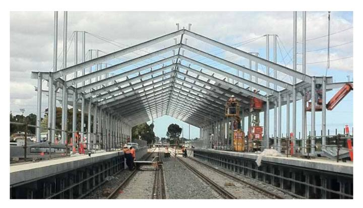
They said the winning Korvest Galvanisers entry scored highly on its market development potential and technical innovation by demonstrating that a high quality hot dip galvanized (HDG) coating can be applied to oversize assemblies without coating blemishes or distortion.
