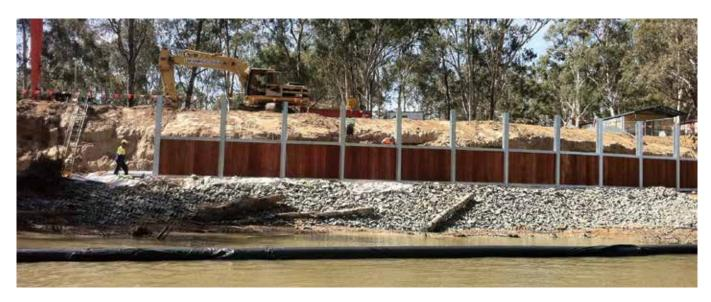
An engineered retaining wall supported by a galvanized steel frame is keeping land subsidence from encroaching on the picturesque Murray River and locals safe from floods whilst allowing red gum timber panelling to reflect the region's treasured tree life.
